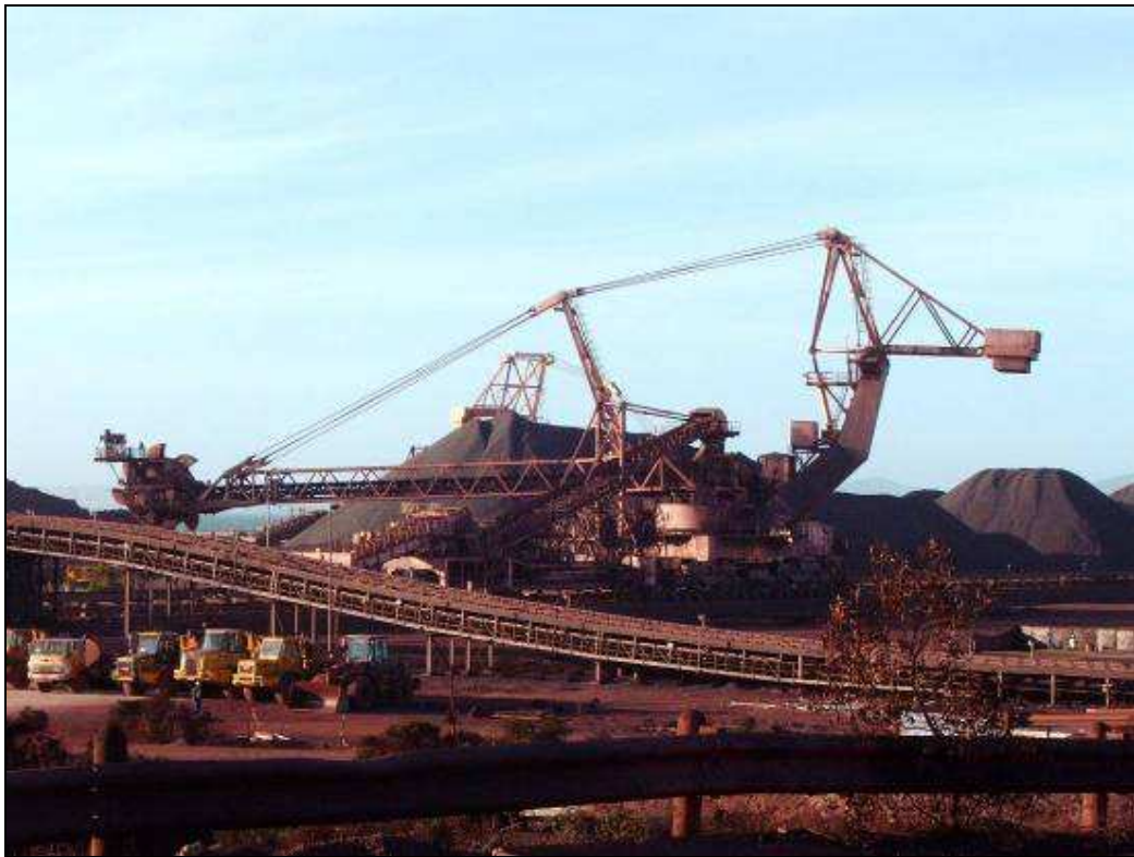
Photo Plate 2: One of the three existing Stacker Reclaimers with associated conveyors.
